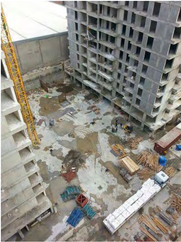
The “4 Towers” construction site in Ankawa.
